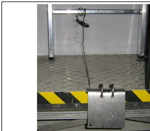
3. Open the door of the car cabin and place the edge protection plate on the bottom edge of the car cabin (to prevent falling).
